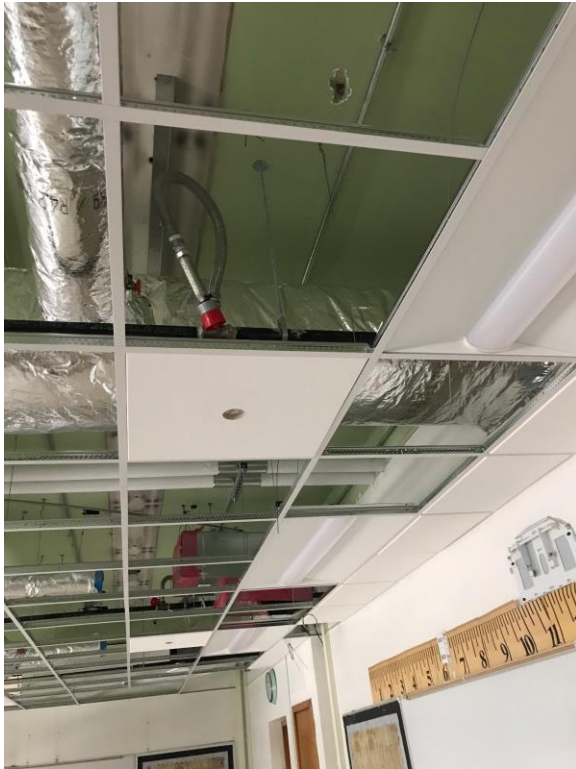
Sprinkler Head Ceiling Tile
